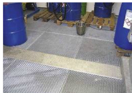
If a drum develops a leak, the chemical drips into the sump tray installed underneath the store
